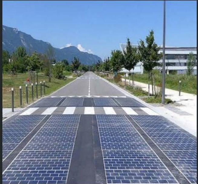
Kaynak: Solar roadway test installation in Savoie, France, Florian P epellin/wikimedia commons
